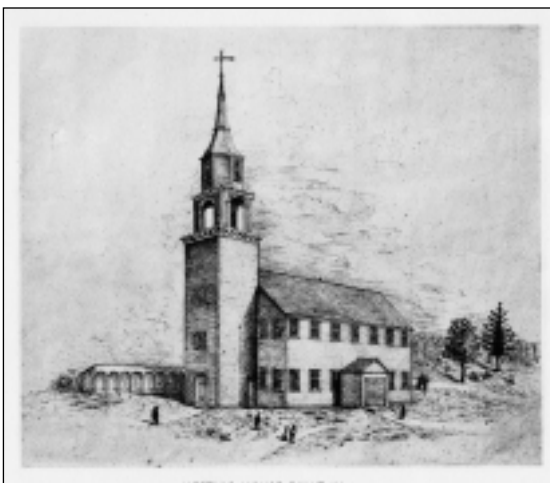
The 1774 Meeting House, showing the steeple that was erected in 1811.
